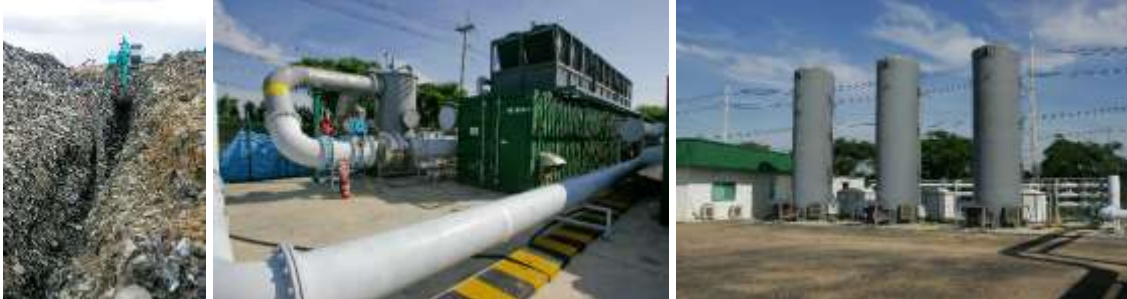
Landfill Gas to Electricity Project
