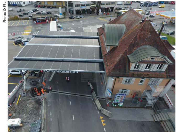
The new roofing with integrated photovoltaic system at the customs post in St. Margrethen.
